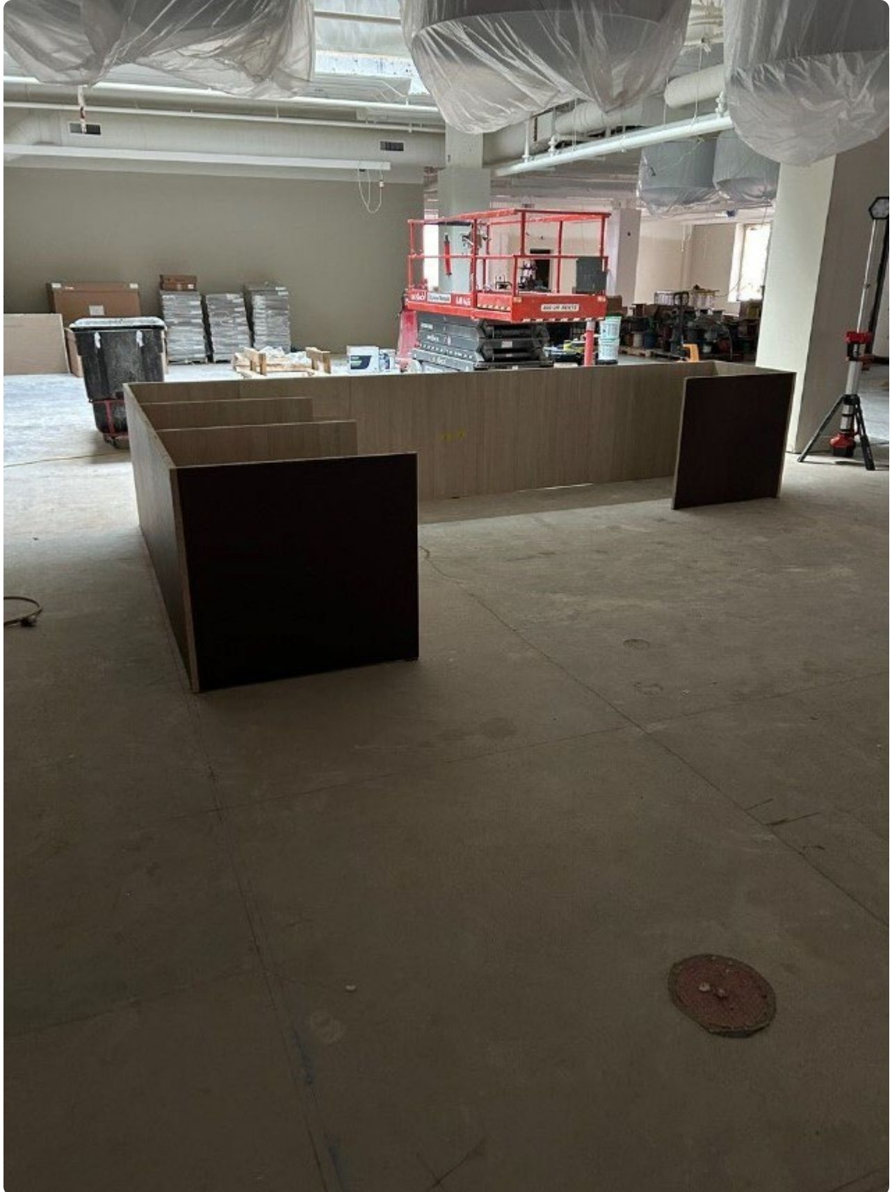
Ground Level Service Desk Installation
