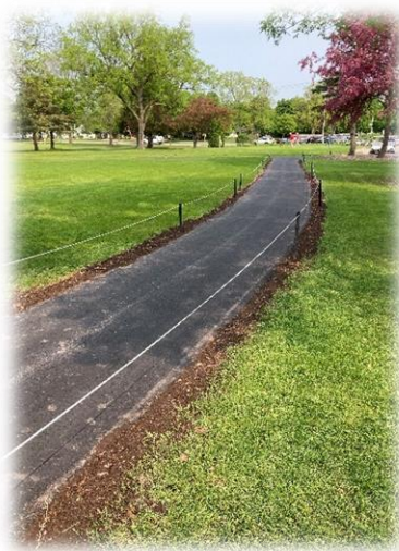
#1 tee path paved and restoration completed waiting for germination.
