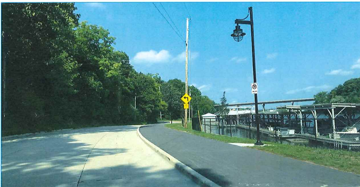
Figure 1 - Lutz Park Multi-Use Trail (as constructed)
